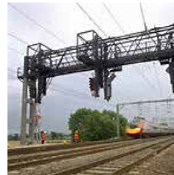
Signal gantry with OLE portal system in background
