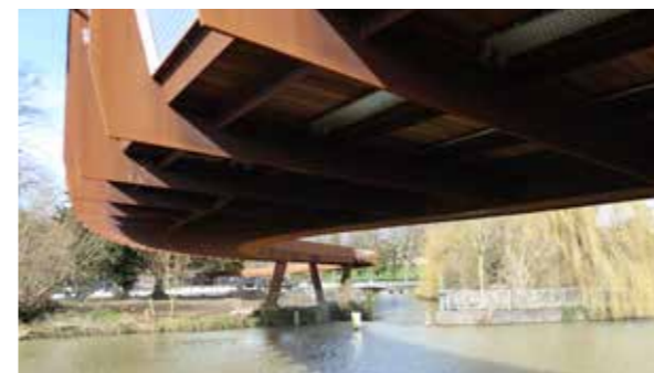
No maintenance Corten structure on 180m long footbridge; University of Northampton, Waterside campus
