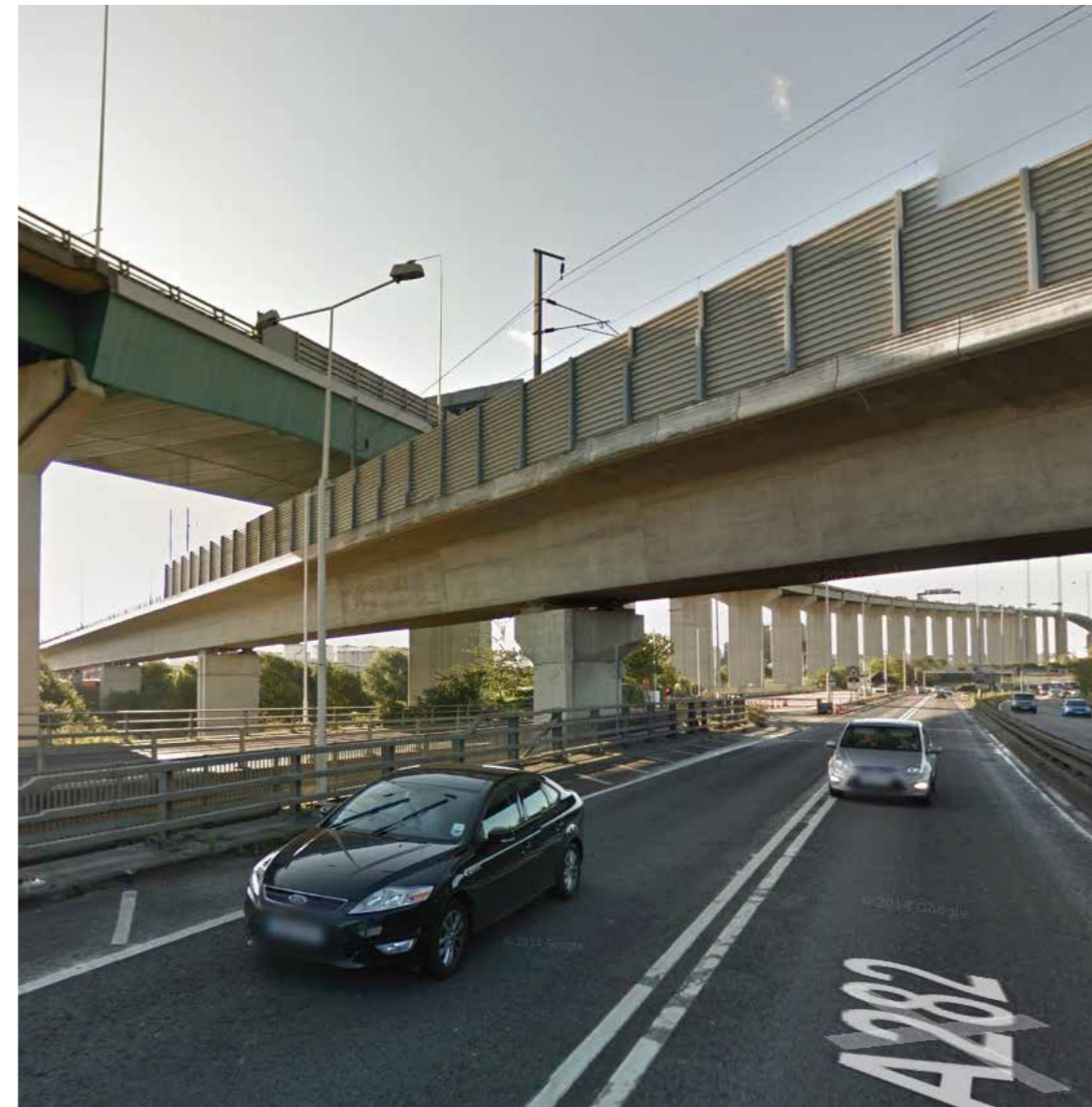
Noise mitigation at the cost of visual intrusion, HS1 crossing the M25, Thurrock
