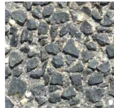
Abutments: Exposed dark coloured exposed aggregate concrete
