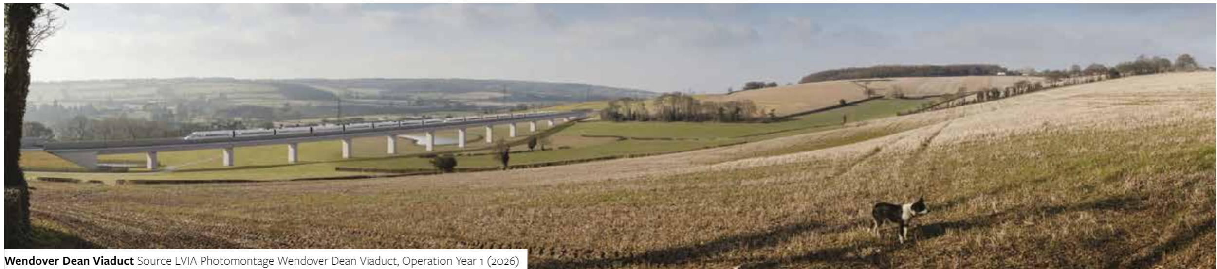
Wendover Dean Viaduct Source LVIA View from King's Lane: Current baseline (2013)
