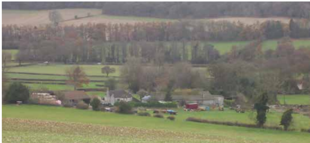
Durham Farm and the immediate context of the proposed Wendover Dean Viaduct. The farm will be demolished.
