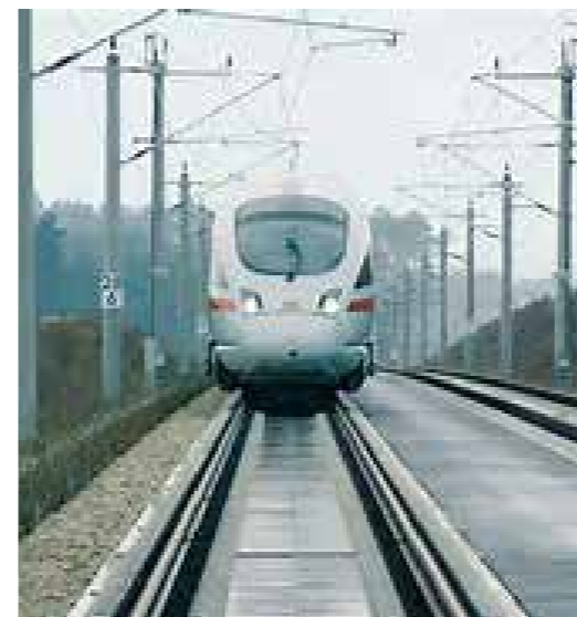
Cantilever OLE masts
