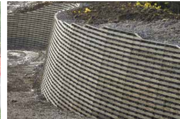
Cribblock foot of slope barrier
