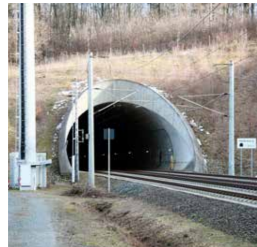
Hellenberg Tunnel, north portal (Germany)
