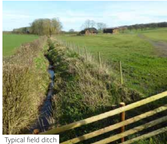
Typical field ditch
