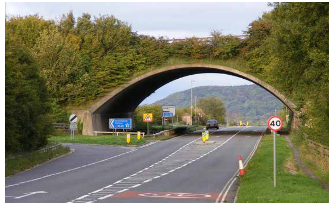
Local example of a 'greened' overbridge on the M40 at Lewknor
