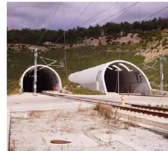
Le Perthus Tunnel, France. Note short porous portal
