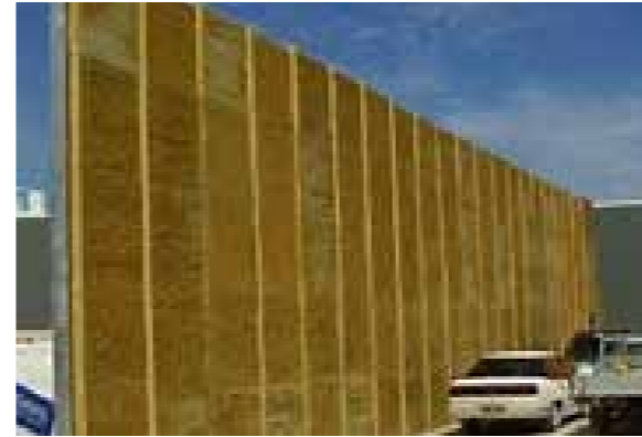
High timber, vertically clad
